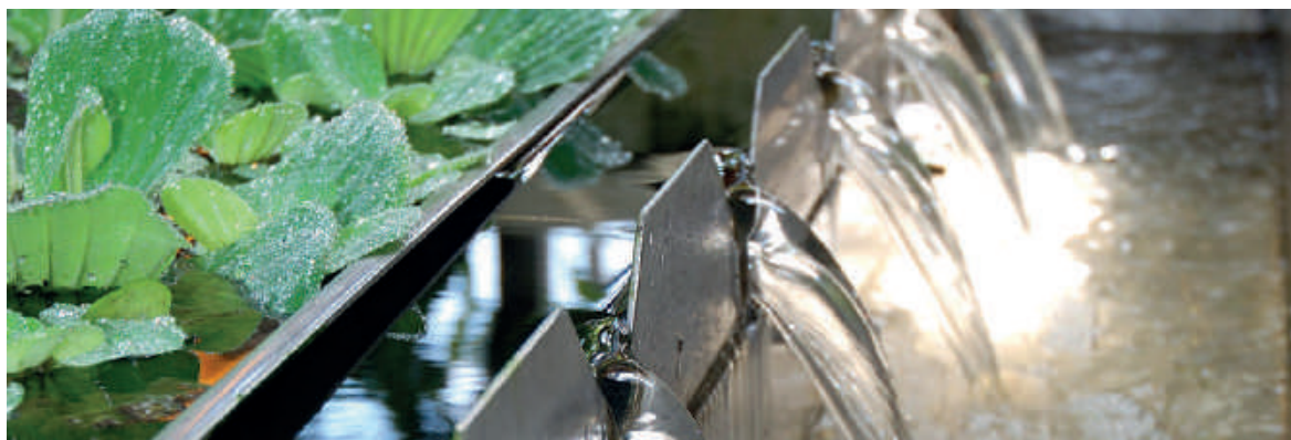
Part of a low-energy wastewater treatment system based around a cascade of biological stages. Biofilms of microorganisms, some living on plant roots, remove nutrients from the effluent. Photo: Organica
