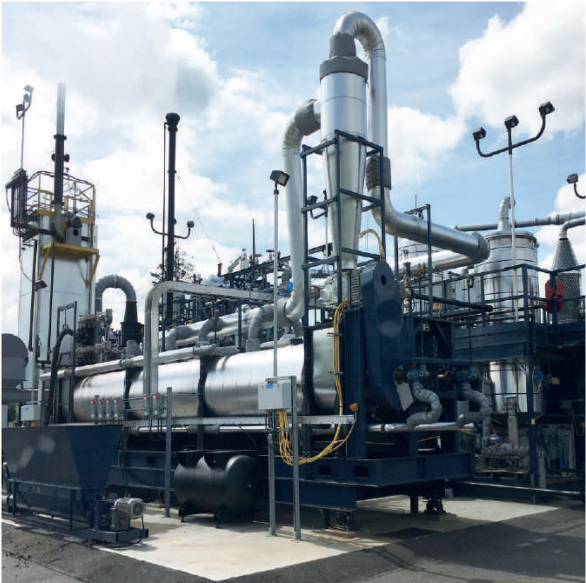
A combined heat and power plant that recovers energy (heat and electricity), potable water and ash from faecal sludge and other combustible waste. Photo: Flickr / SuSanA Secretariat / Janicki Bioenergy
