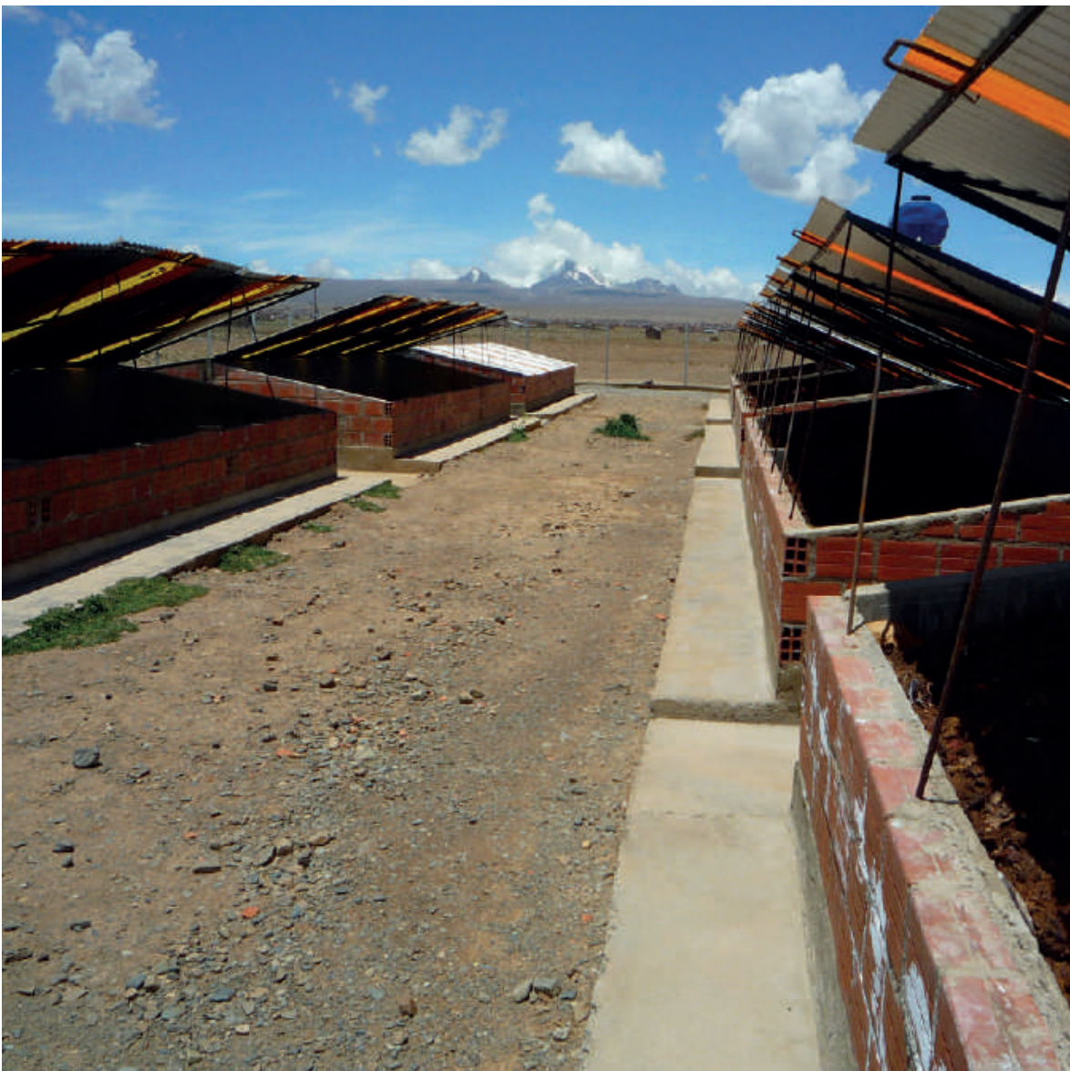
Faeces composting for agricultural reuse in a project in El Alto, Bolivia. Urine and faeces are collected separately using urine-diverting dry toilets. Greywater is applied to household constructed wetlands. Photo: Kim Andersson
