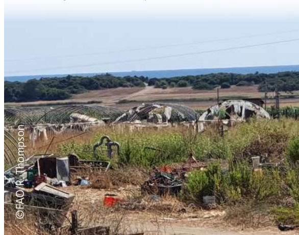
Abandoned greenhouses, Italy.
