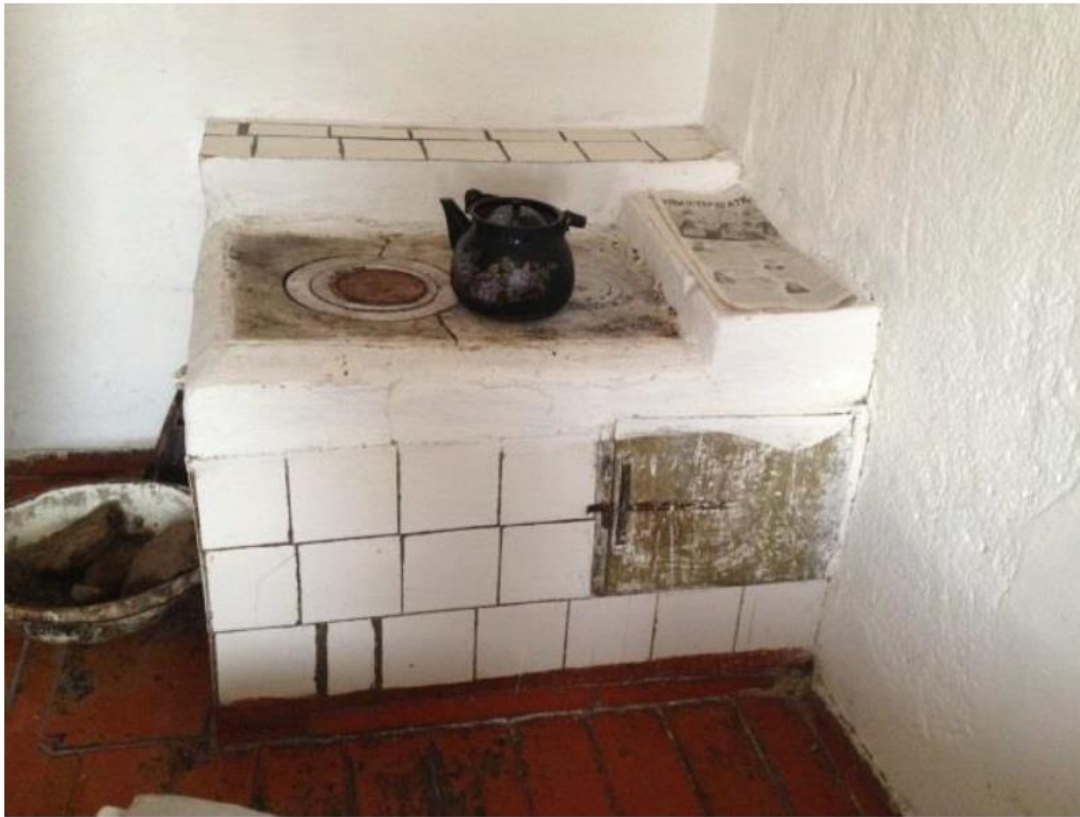
Figure 29: Typical solid fuel masonry stove used for heating and cooking in Kazakhstan
