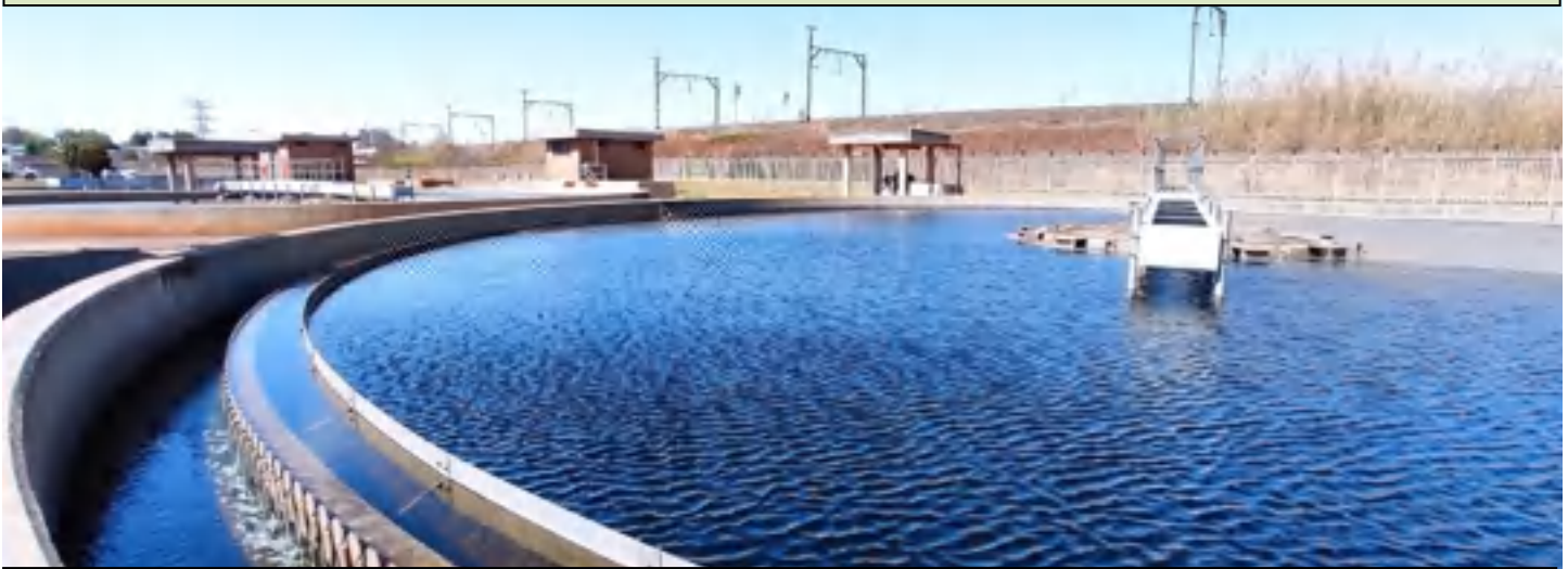
Technical Site Inspection score of 96%. No words required. This final effluent captures the excellent operations which is a characteristic of the JP Marais WWTW. This final settling tank will not look out of sorts at any potable water treatment plant, showing excellent final water quality, level weirs, clean surface and a working walkway.
