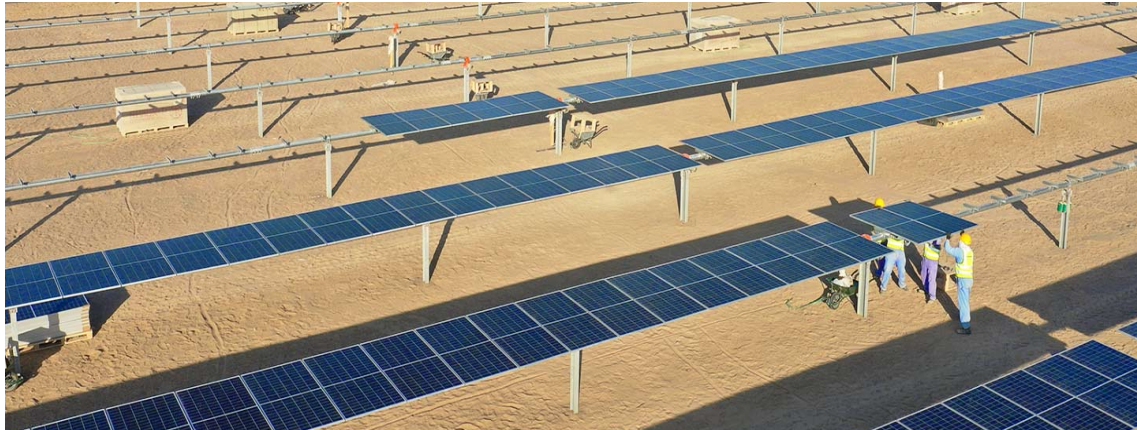
Workers installing one of 1.4 million solar panels that make up the Ibri II 500-megawatt solar photovoltaic independent solar power plant, the largest utility-scale solar park in Oman. Photo © AIIB 2021
