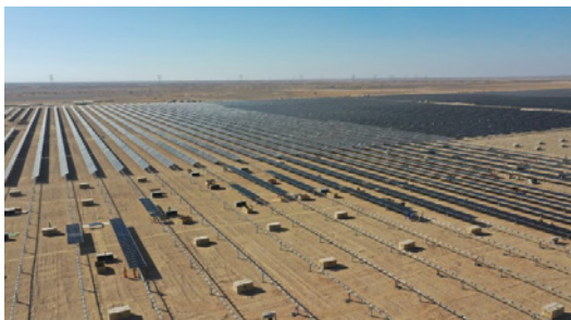
The Ibri II 500-megawatt photovoltaic independent solar power plant in Oman. Once finished, the plant will cover 13 square kilometers. Photo © AIIB 2021
