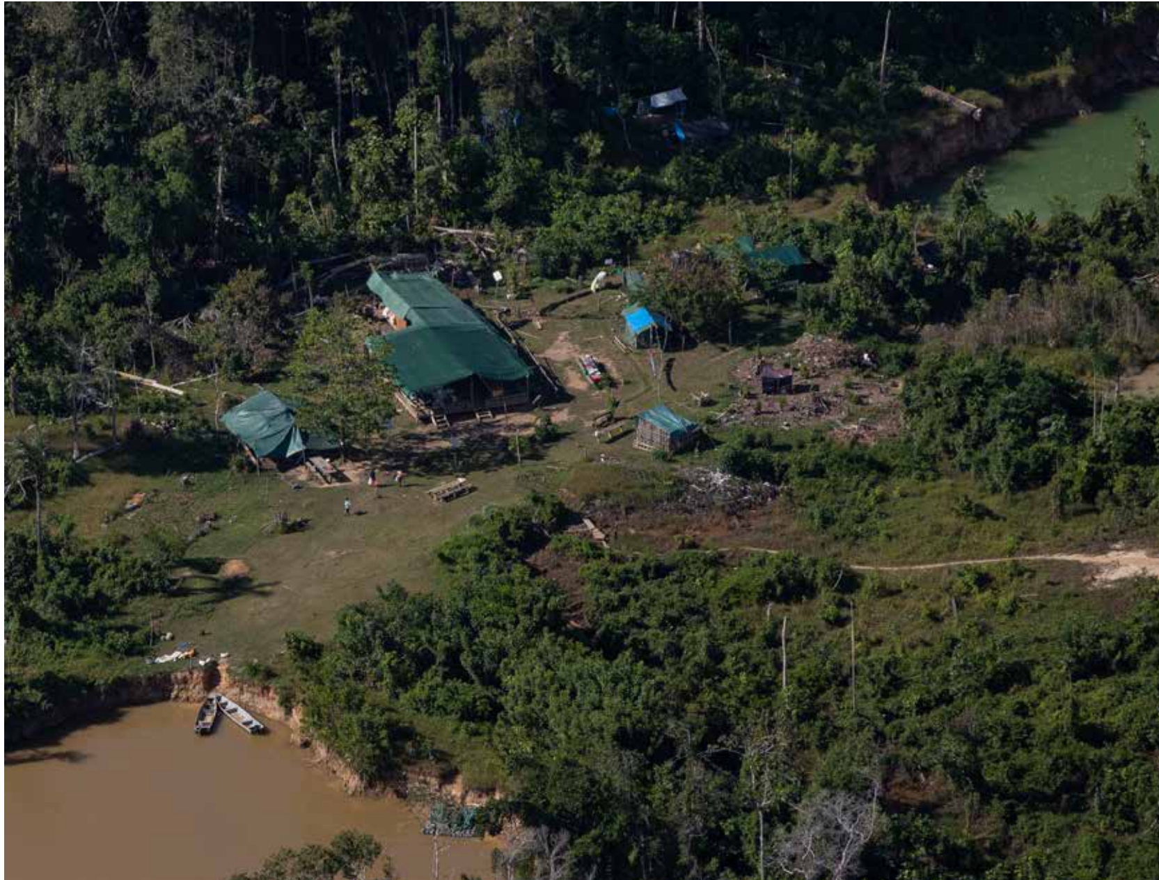
Photo 6: Structure that supports the mining logistics in the Uraricoera.
