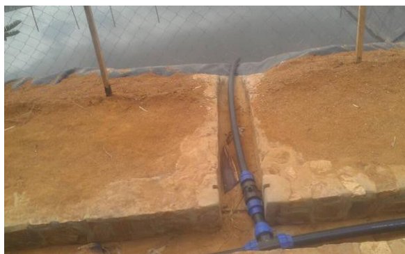
(b) Drip kit connected to a small water reservoir created with dam sheetting.
