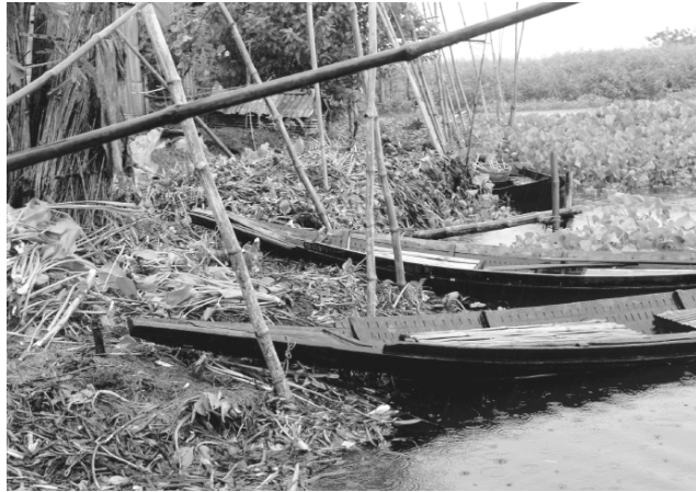
Water hyacinth for erosion-proofing in Betgram
