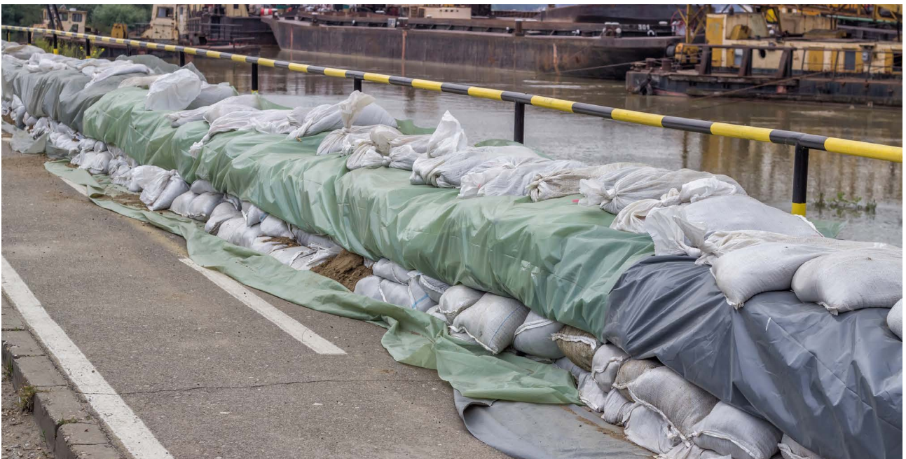
Wall of sandbags for flood defense, sandbag barricaded Photo: iStock
