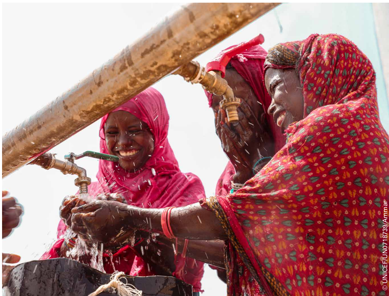
In Ashat village within the Tokar locality in the Sudan, children and adults collect water from a rehabilitated facility that now serves around 350 households. The motorized water system brings safe water closer to families who previously walked 4 km across a valley to access it—transforming daily life in Gorora and Tokar localities.
